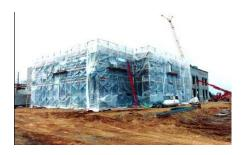
addition, the minimum temperature of (both surface and ambient temperatures) must be maintained until all the layers and components of the EIFS assembly have cured, usually 24 to 48 hours after completion of each phase of work (i.e., base coat, finish coat, etc.). Ensure any required mixing of EIFS components conducted within the same temperature quidelines the individual components.
